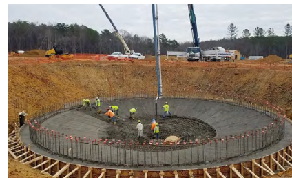
The conical foundation of the thickener tank is poured using a pump and dozens of truckloads of ready-mix concrete from supplier Wayne Davis Concrete. The ready-mix firm premixed Xypex Admix C-500 in each truck using 15-lb water soluble bags.
