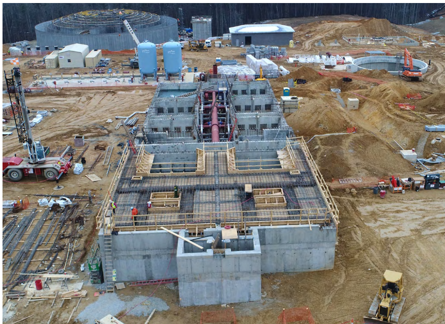
The conical foundation of the thickener tank is poured using a pump and dozens of truckloads of ready-mix concrete from supplier Wayne Davis Concrete. The ready-mix firm premixed Xypex Admix C-500 in each truck using 15-lb water soluble bags.
