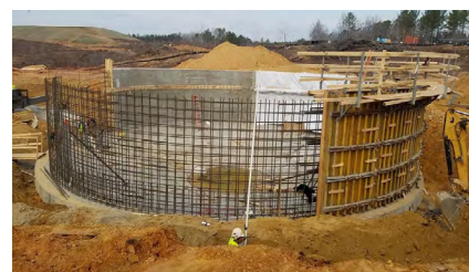
The walls of the thickener tank, used to condense the volume of residual solids, are reinforced, formed and poured.
