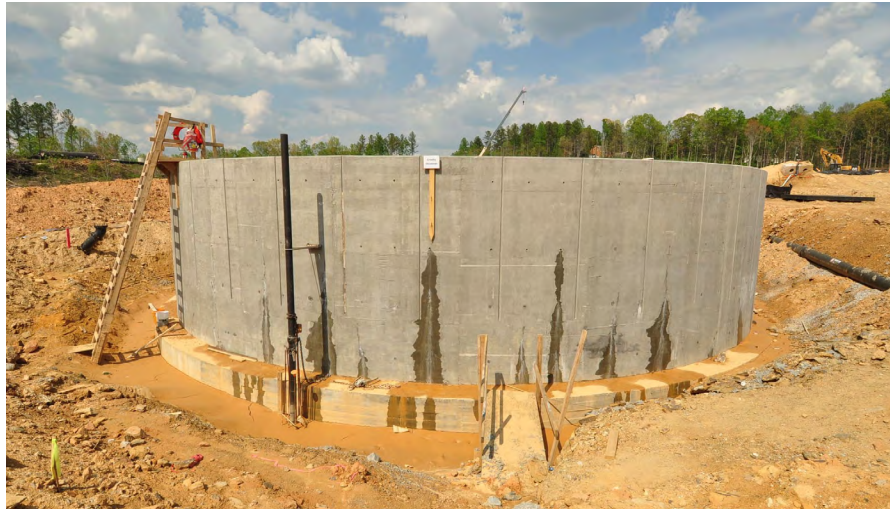
Photo taken April 13, 2017 at an early stage in leak testing.
