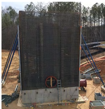
Extensive steel reinforcement is built prior to pouring the walls of the clearwell splitter box.
