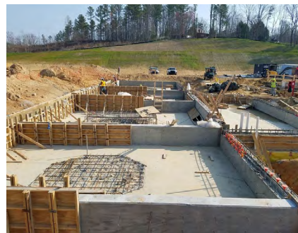
Chemical storage building foundation takes shape. Exterior containment walls are formed and poured using concrete treated with Xypex Admix C-500.
