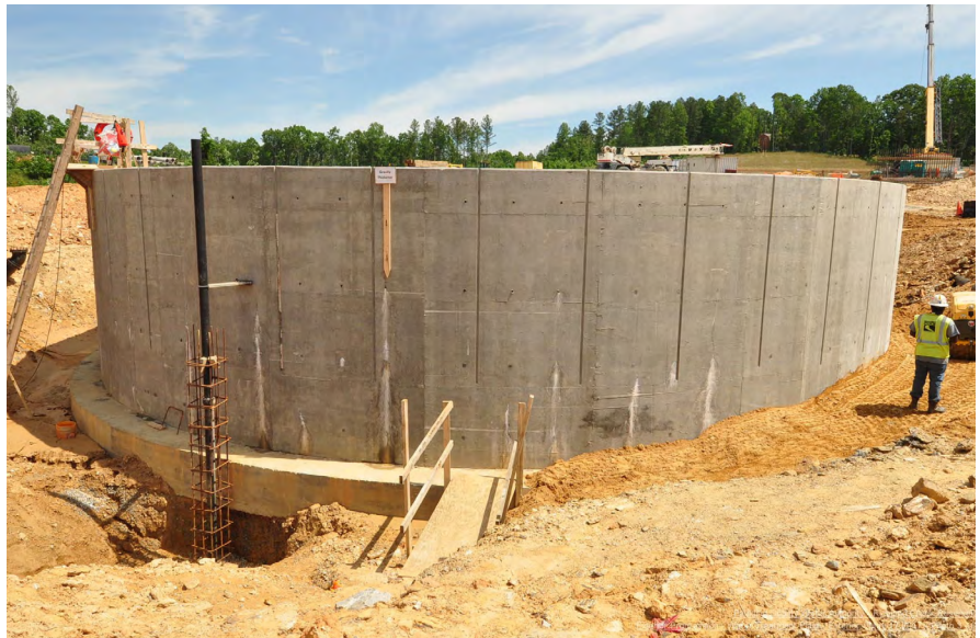
May 17, 2017. All cracks have been sealed by Xypex Admix and the contractor has begun to backfill the tank. No crack injection or crack patching was required in the thickener tank or any other WTP structure thanks to the incorporation of Xypex Admix in the concrete.
